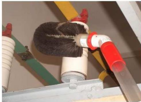
Fig. 18 and 18a: Circular brush H091-07
