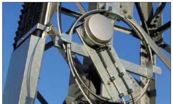
Example of OPGW installation
