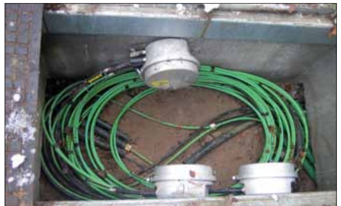
Manhole installation with T240 closures
